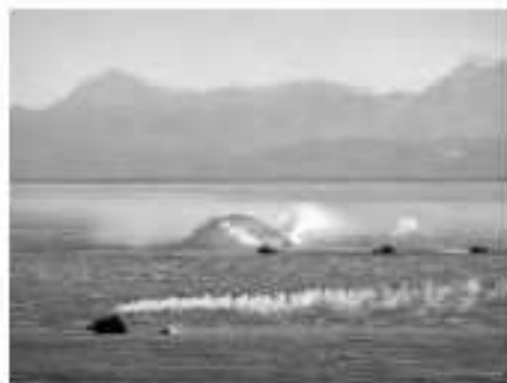
Smoothing snow at McMurdo Sound to prepare for aircraft landings.
